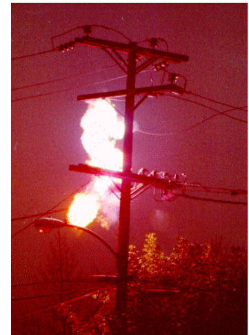
Shorted power line causes arc
