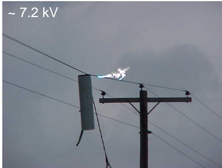
Shorted power line causes arc
